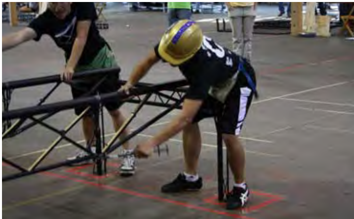
Above, below: The University of California at Davis design included several custom tools for holding members in place and making connections, shown below in the staging area and above in use during construction.
