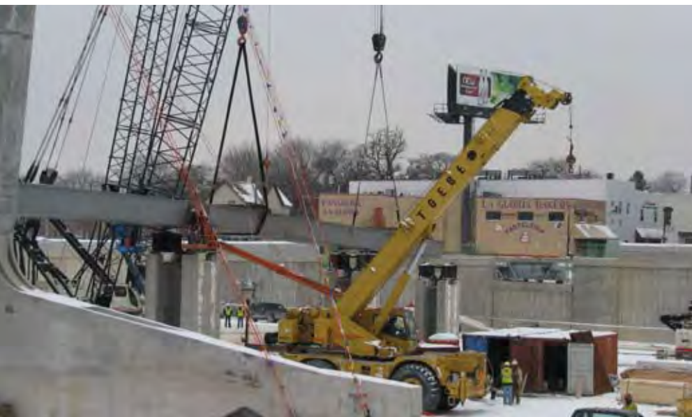
The complex erection sequence required the use of three falsework towers, which supported the west span until the cable stays were attached.
