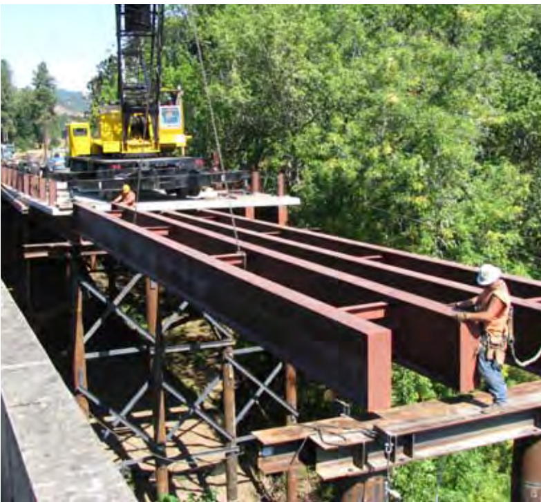
▲ The North Umpqua River detour bridge being constructed adjacent to the existing bridge. The steel girders for the 120-ft main span were salvaged and modified from a local bridge replacement.
