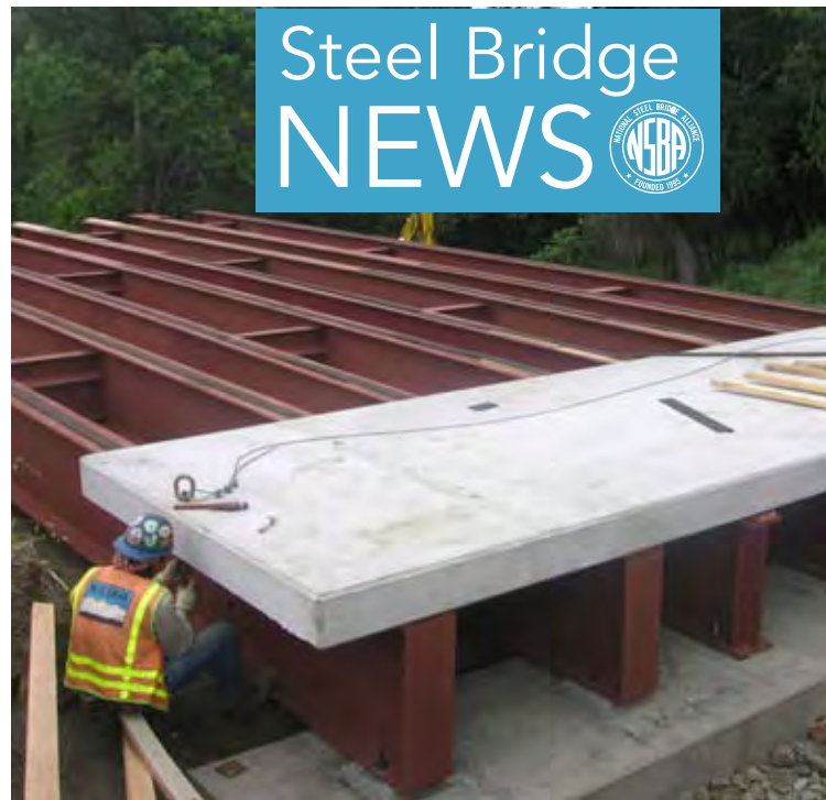
▲ Workers install the precast concrete panels that make up the deck of the temporary North Umpqua River detour bridge. Douglas County plans to reuse the deck panels and steel bridge rail at different sites after the permanent bridge is complete.
