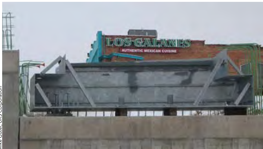
The west abutment prior to setting the tub girder. Note the non-symmetrical support system, with hold down anchorage on the left and bearing on the right.
