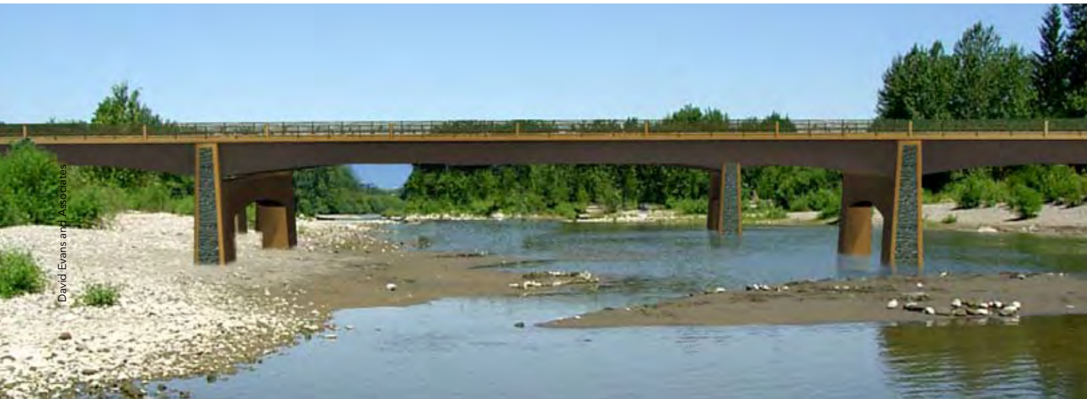
▲ The new Sandy River bridges will feature rock facade treatments on the bridge piers, abutments and decorative pylons consistent with the Interstate 84 Corridor Strategy aesthetic design guidelines.
