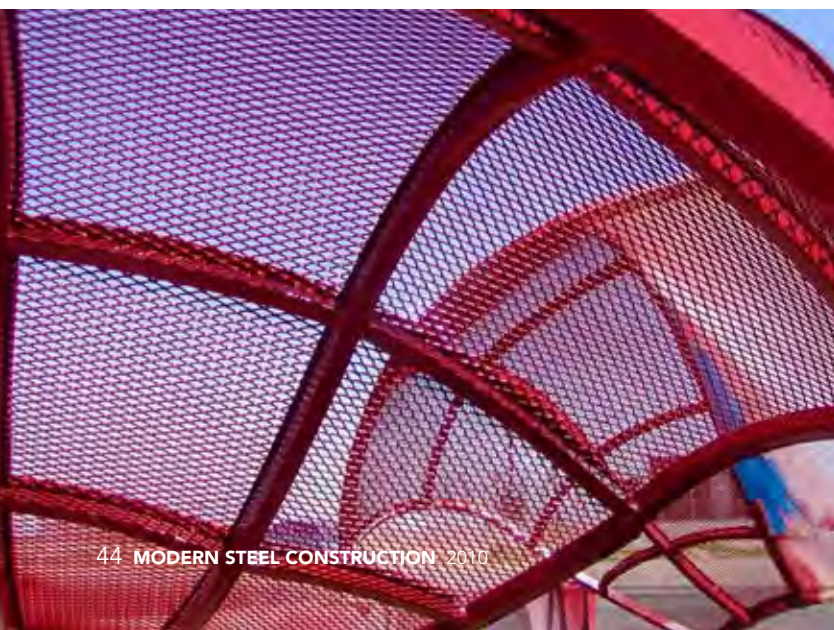
Below: Each piece of wing consists of several expanded metal sections, which required that workers be careful when welding it to the structural members to avoid damage from excessive heat.
