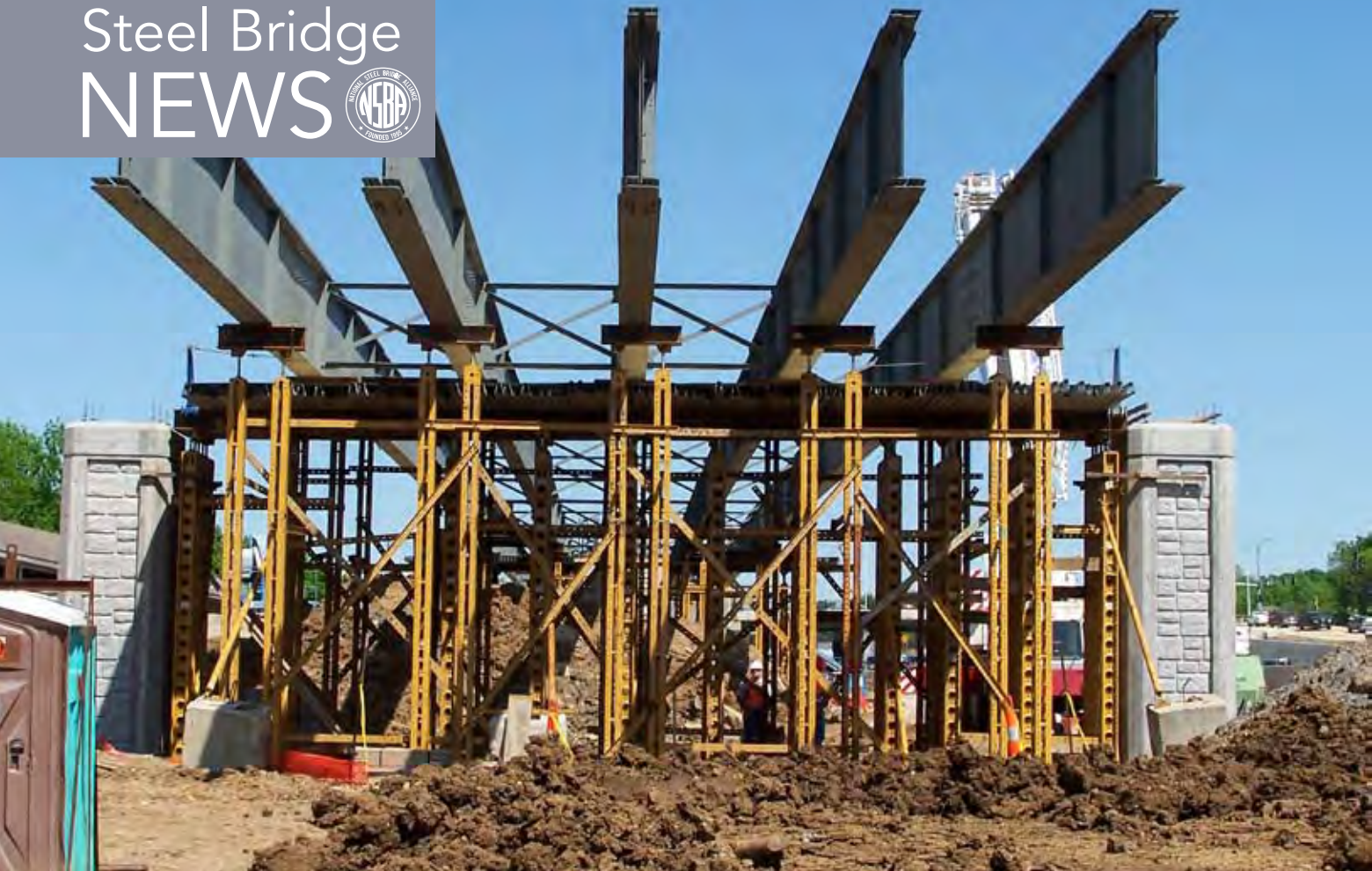
▲ ▼ The steel girders were supported by falsework (above) until the concrete cap beam was cast and cured and post-tensioning was completed.
