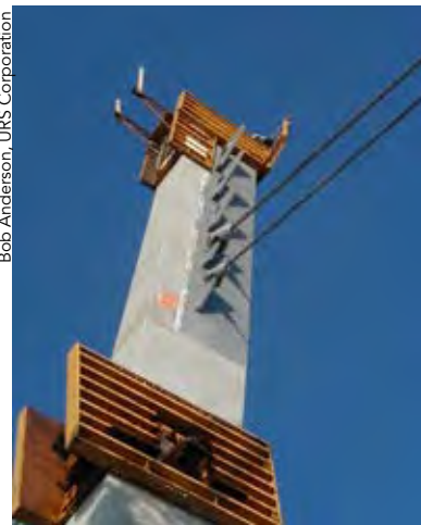
The pylon stay cable housing in place with the lower two back stays attached.
