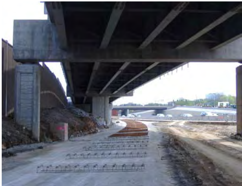
▲ To reduce the height of the bridge by several feet, the steel I-girders were framed in with the concrete cap beams at three of the four interior piers.
