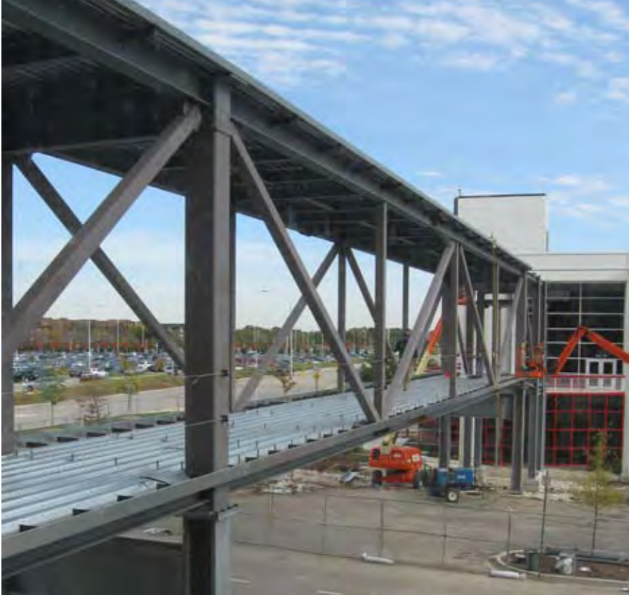
Architecturally exposed HSS sections form the verticals and diagonals of the trusses on this bridge linking the Health Careers and Natural Sciences building to the student union at the College of DuPage.
