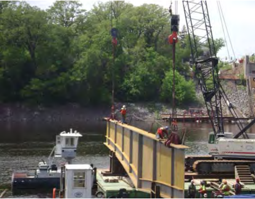
left, top: The haunched section of this interior girder shows the longitudinal stiffeners that were required at the river piers.
