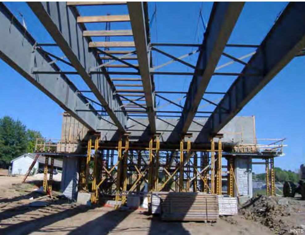
▲ ▼ The steel girders were supported by falsework (above) until the concrete cap beam was cast and cured and post-tensioning was completed.
