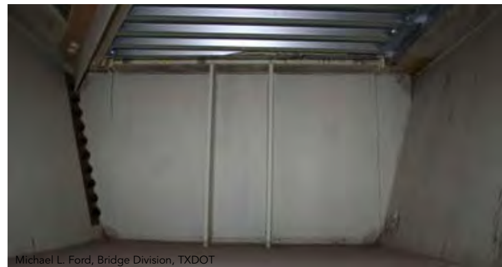
Fig. 6: Internal diaphragm.
